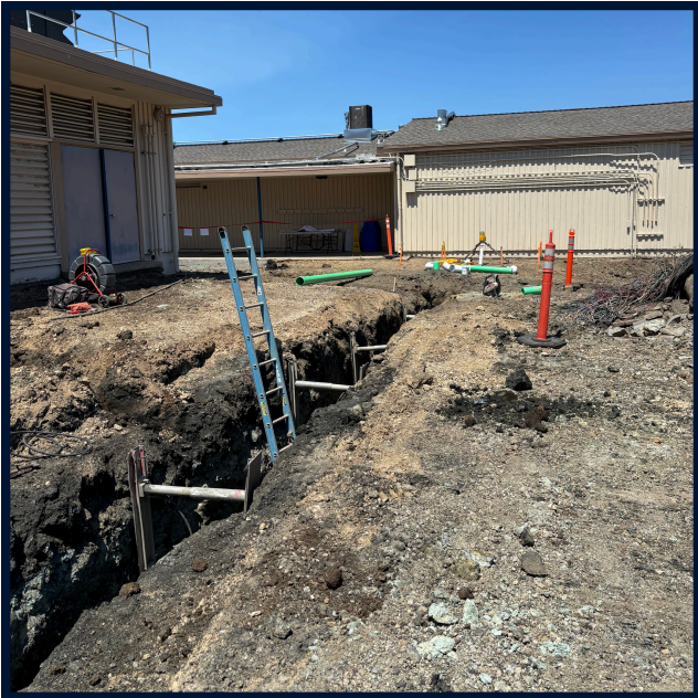
Pictured above are trenches for the underground utilities.
